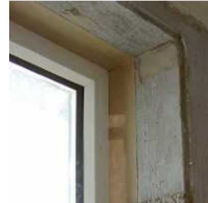
Fig. 3. 22 – The sealing tape, on which plaster can be applied, will then link the interior plaster and the window
